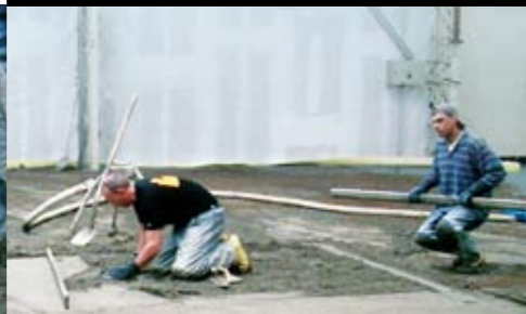
2 Spreading the screed to the specified height
