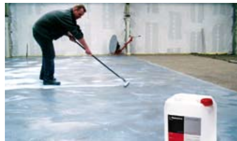
5 An evaporation protection agent (e.g. Meboplast diluted 1:2 with water) is applied once the screed can be walked on
