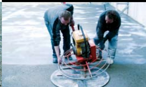
4 After scattering the hard aggregates, these are smoothed into the still-fresh surface using a power float
