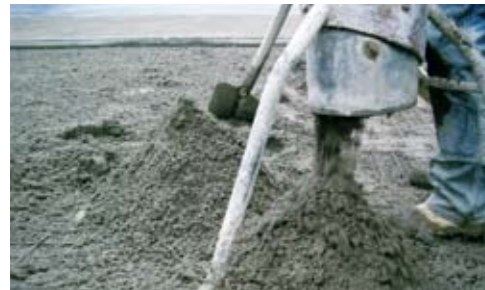
1 Placement of a cementitious screed as an industrial screed
