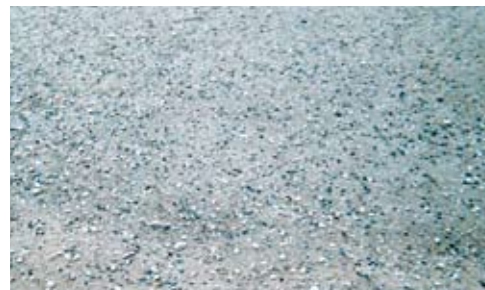
3 Screed surface with scattered on hard aggregate (hard aggregates according to DIN 1100)
